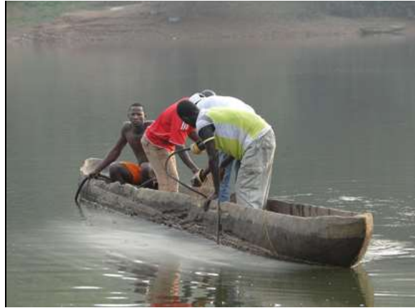
Repair of the broken cable of the ferry
