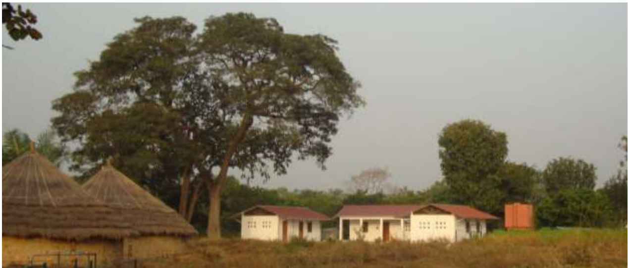
Casa Daridibó with to the left the back side of two bungalows of the Fonda Huuwa camp site
